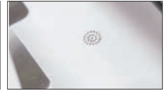
Each compartment has a floor drain for quick drying after cleaning.
